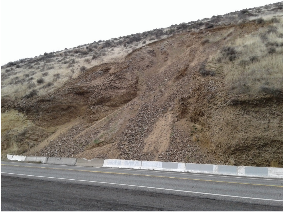
Figure 24. Dry ravel and headward recession of Yakima River Canyon slopes. Near Milepost 18. Source: Karl Lillquist, March 2018.
