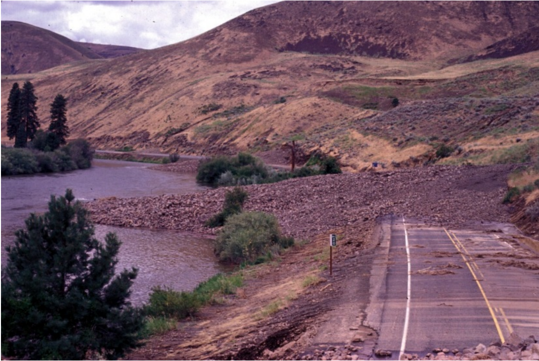
Figure 22. View up canyon at Milepost 20. Source: Karl Lillquist, 4 July 1998
