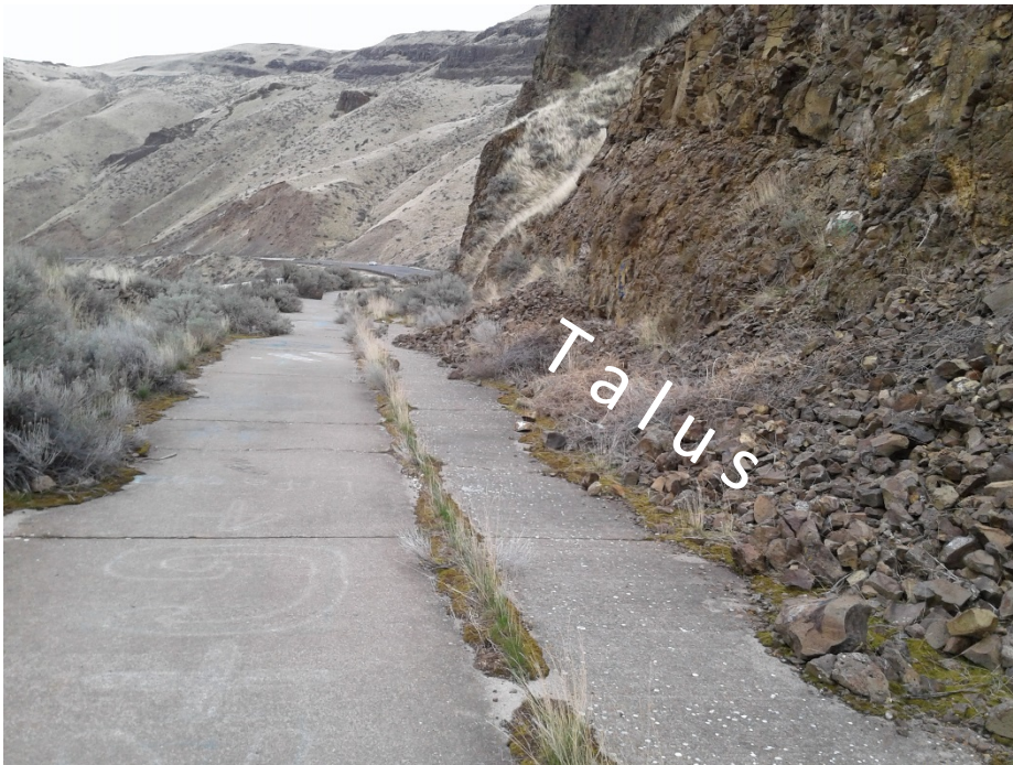
Figure 27. Talus accumulation on old US 97, south end Yakima River Canyon. Source: Karl Lillquist, March 2018.
